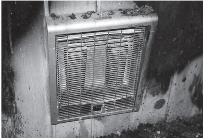
**Figure 1-14** This aging wall heater was the cause of the fire in this home. As a restoration contractor, you'll be dealing with fires of all sizes and types.
