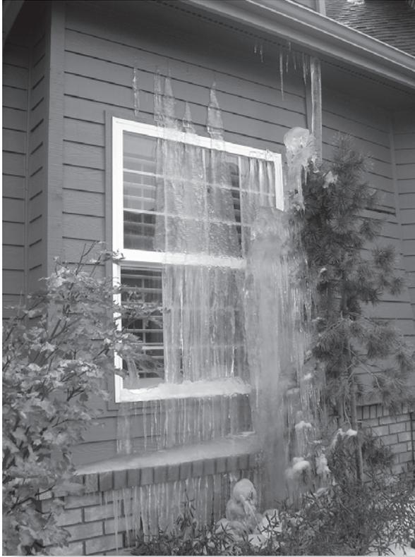
**Figure 1-13** A broken pipe on a second floor caused a massive water leak in this home. The water eventually made its way into the exterior walls and behind the siding, resulting in this rather dramatic ice sculpture in the front yard.
